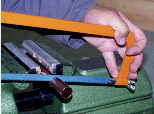
1. Rectangularly saw off the pipes
